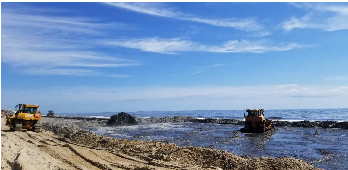
Figure 5.1. Example of beach fill being constructed (Carolina Beach, 2019).
